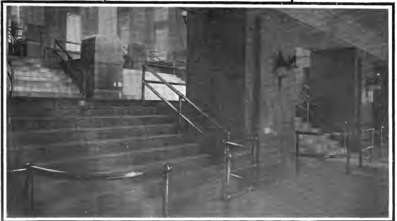
(Upper) Exterior view of New Grand Central Palace. (Lower) Grand stairway leading from street level to main floor
